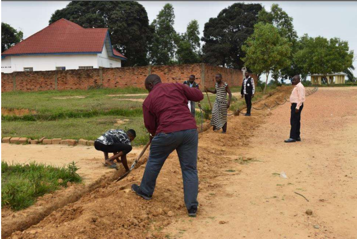
Digging a trench for the water line to the school
