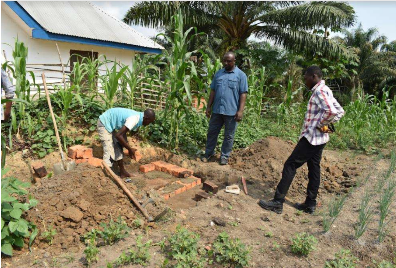
Preparing the water fountain and faucet near the school 4
